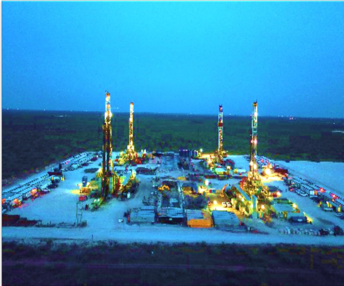
8 WELLS DRILLED BY 4 RIG PAD – FELIX ENERGY
